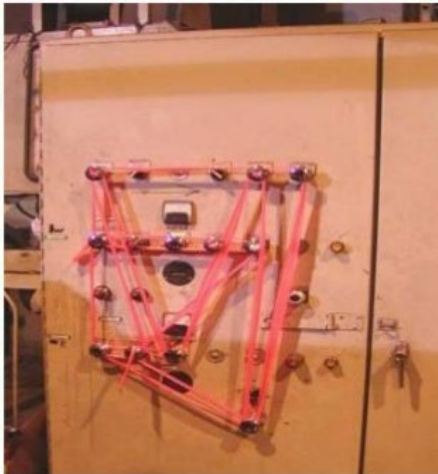
Example of a bad lockout/tagout
